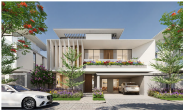
4 BEDROOM STANBALONE VILLA TYPE - C STREET VIEW
